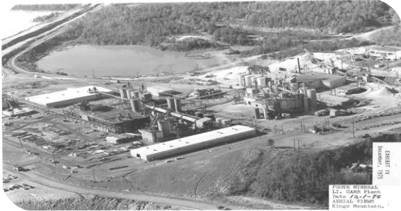
Spod Conversion Plant (Kings Mountain, NC)
